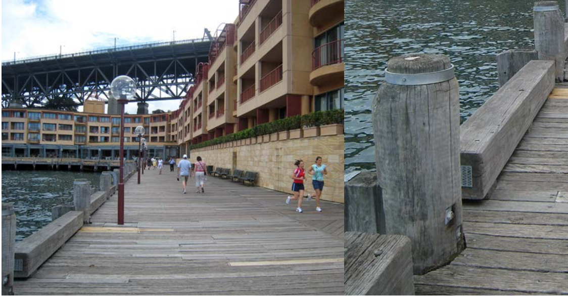
ABOVE: Timber promenade adjacent to hotel RIGHT: Bollards and fenders
